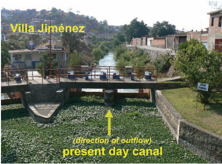
Figure 14: Canal at Villa Jiménez (Stop 3) that served for draining Zacapu lake more than 100 years ago (direction of the outflow is indicated by arrow).
